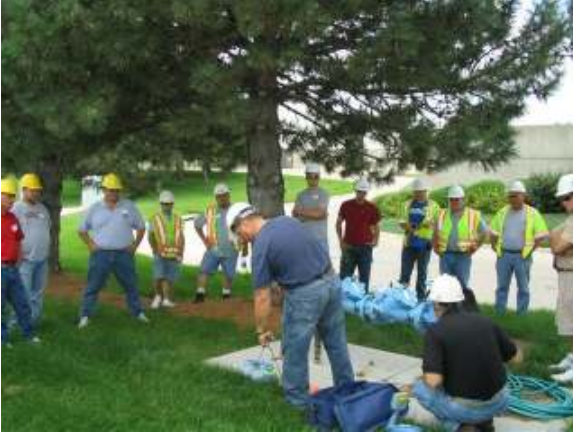
Workshop Instructor, Travis Beran with Subsurface Solutions conducts hands-on water line training.
